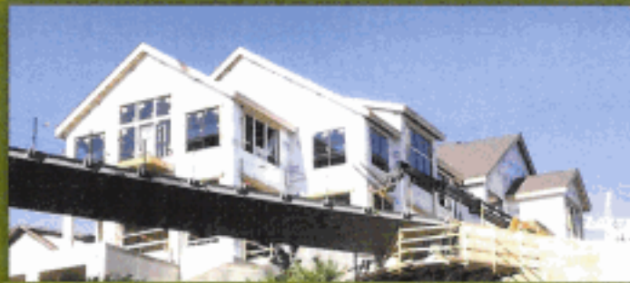
The new $23M Bridge Park footbridge under construction
